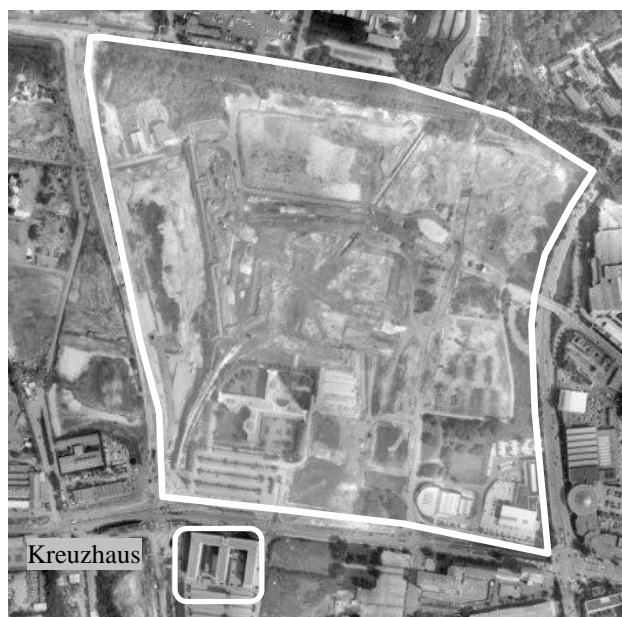
Figure 1. The main excavation area Site
